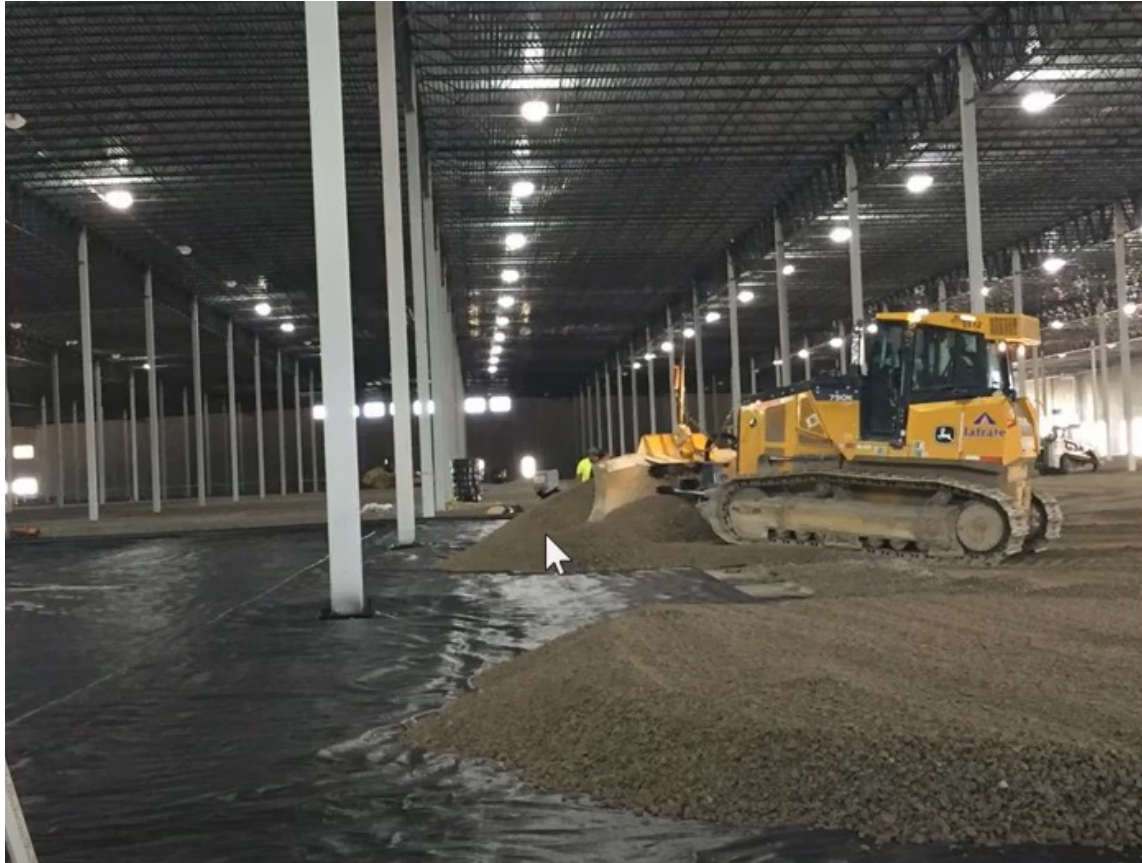
GEOTEXTILE FABRIC & PROTECTION LAYER INSTALLED
